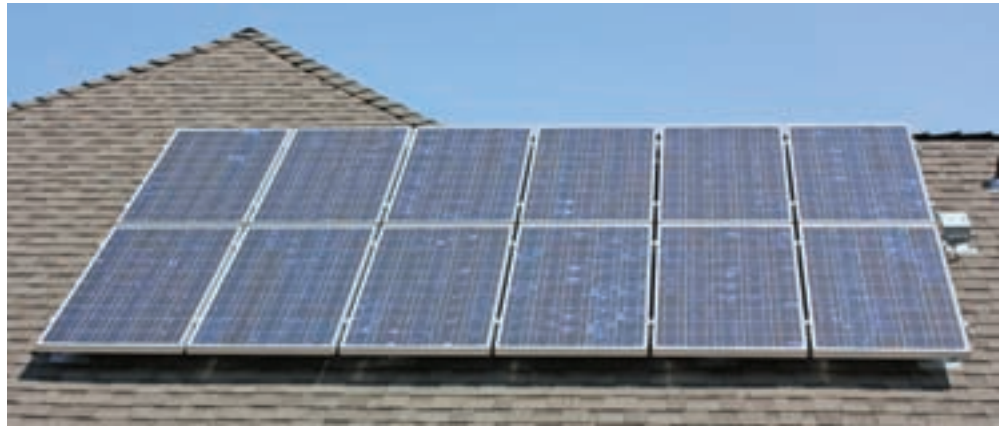
PV systems are great additions to any home with good solar access, but their efficiency is still well under 20%. Payback time on PV systems can be many years.
