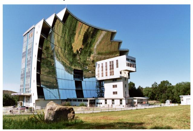
A solar furnace is a structure used to harness the rays of the sun in order to produce high temperatures, usually for industry. This is achieved using a curved mirror (or an array of mirrors) that acts as a parabolic refector, concentrating light (Insolation) onto a focal point. The temperature at the focal point may reach 3,000° C (5,430° F), and this heat can be used to generate electricity, melt steel, or make hydrogen fuel.
